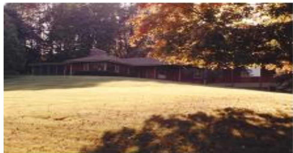
Collins Family Home in Cedar Rapids, circa 1980. Addition with Redwood Siding built about 1954.
